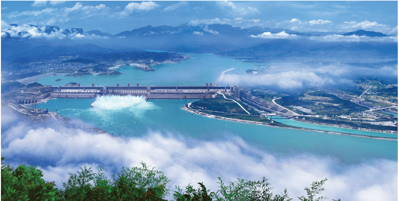
Three Gorges Dam is discharging water
