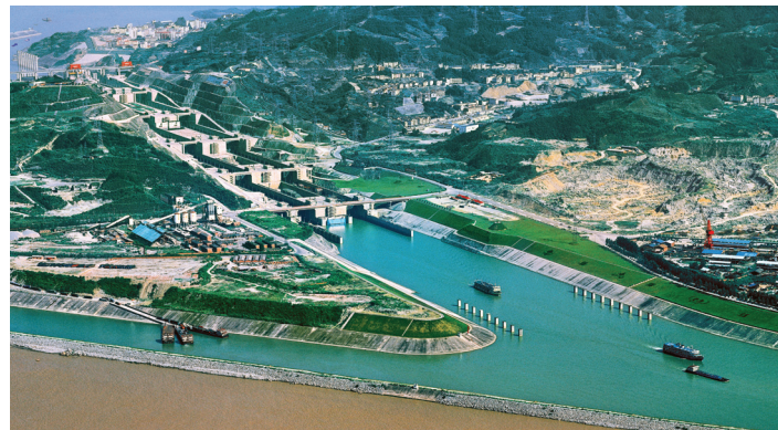
Permanent five-stage ship lock of the Three Gorges Project
