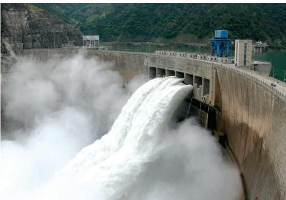
Ertan Hydropower Station in Sichuan Province
