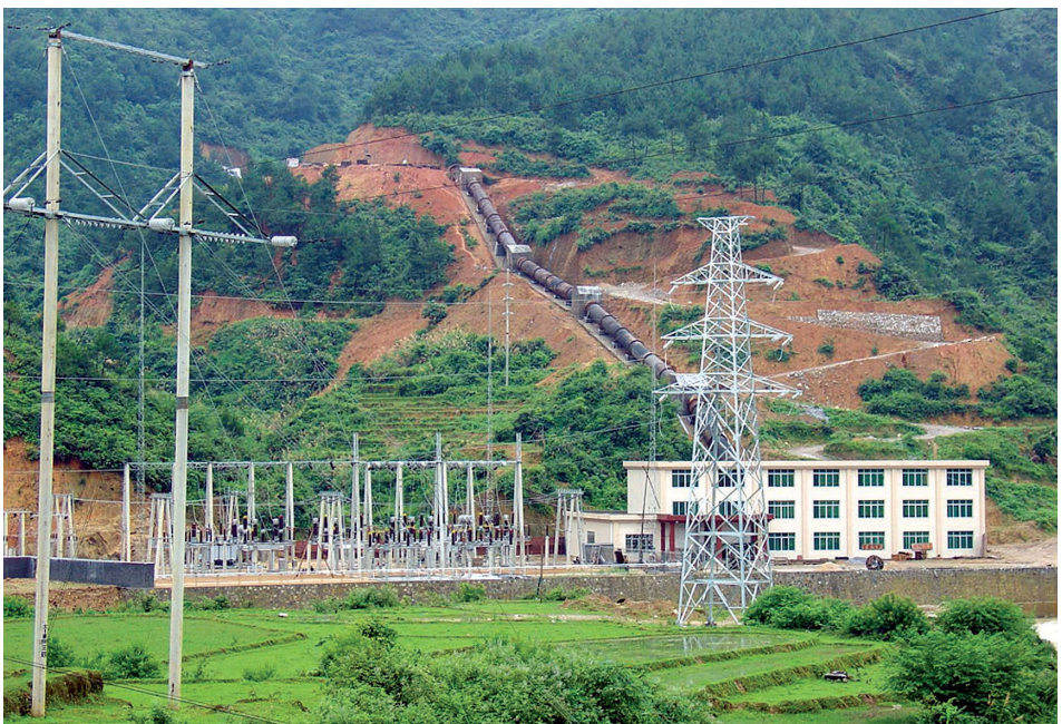
Shimenqiao Small Hydropower Station in Guangxi Zhuang Autonomous Region
